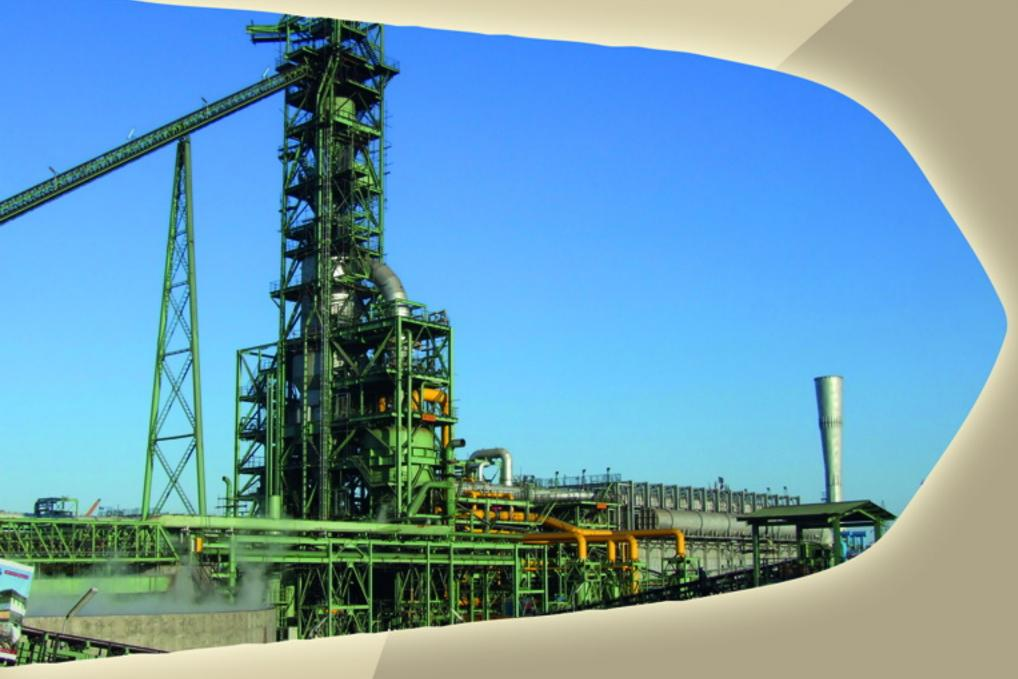
ranian Ghadir Iron and Steel Company (IGISCO) was established in 2007 with an overall production capacity of 800,000 ton per year of sponge iron(DRI). The production process was based on Midrex technology. The plant is located in the central part of Iran close to Ardakan in Yazd province and in an area of almost 90 hectares.
